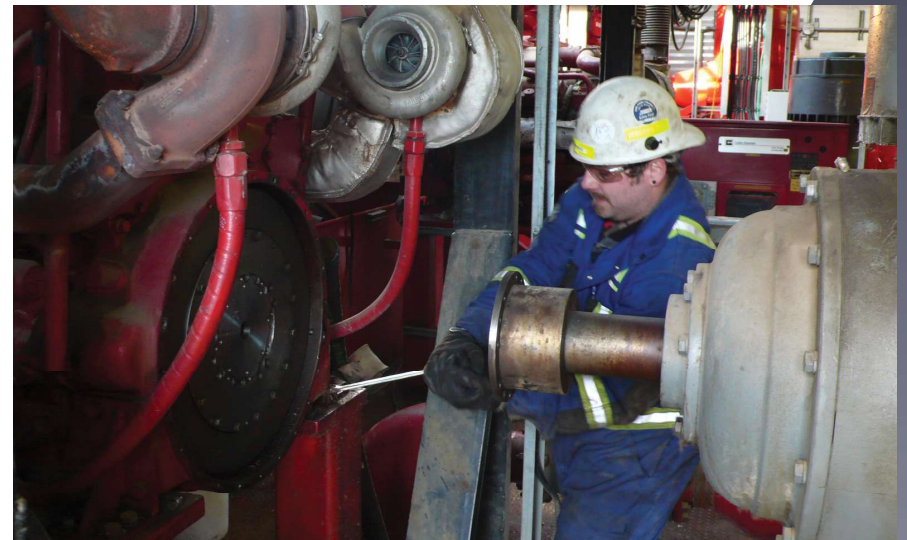
Installation of a fire water pump
