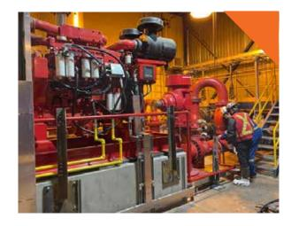
pump-motor (torque) couplings. These components are critical to delivering the expected power to your system, delivering the outputs necessary to keep your assets protected should a fire occur. Unfortunately, over time these components can wear, crack, or in a worst-case scenario, break just when your need your firewater system most.
