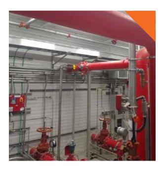
Diaphragm balancing valves are required to have a fluid flush through the diaphragm section with water of foam concentrate until fluid appears clear or new. Diaphragm balancing valves control flow rates in different piping branches to deliver desired flows beyond the valve. Like strainers, these valves can collect debris and buildup over time, so servicing is needed at least every five years.
