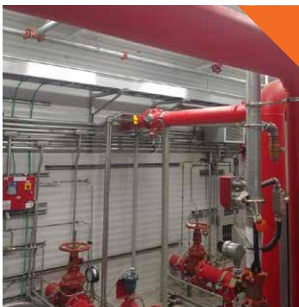
Diaphragm balancing valves are required to have a fluid flush through the diaphragm section with water or foam concentrate until fluid appears clear or new. Diaphragm balancing valves control flow rates in different piping branches to deliver desired flows beyond the valve. Like strainers, these valves can collect debris and buildup over time, so servicing is needed at least every five years.
