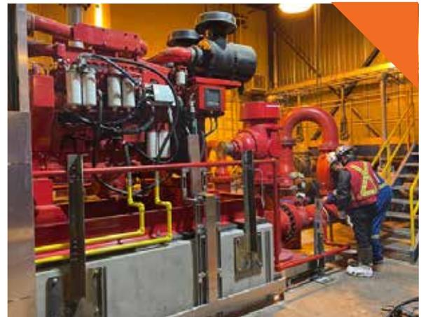
pump-motor (torque) couplings. These components are critical to delivering the expected power to your system, delivering the outputs necessary to keep your assets protected should a fire occur. Unfortunately, over time these components can wear, crack, or in a worst-case scenario, break just when you need your firewater system most.
