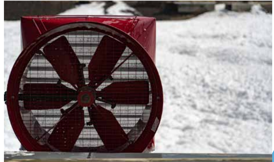
Annual flow testing and inspection of a foam suppression system
