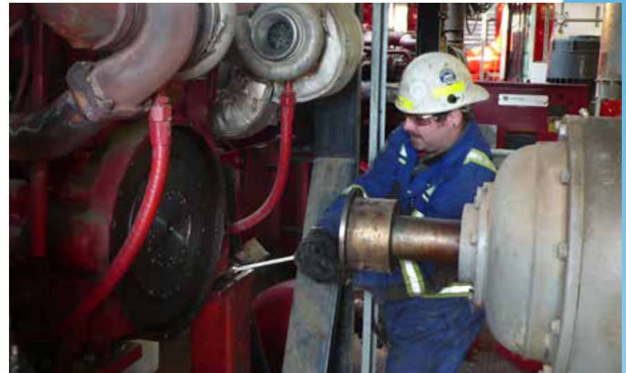
Installation of a fire water pump
