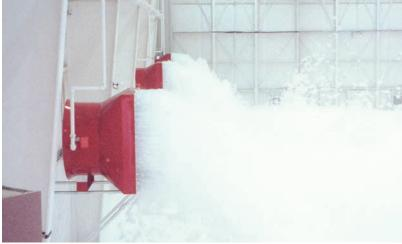
CHEMGUARD high–expansion foam systems provide fire suppression solutions for a multitude of special hazards. The portfoilio offers UL Listed configurations, design flexiblity for utilization of inside or outside air supply, and specific generator models for LNG hazards. All CHEMGUARD high–expansion foam generators are CE Marked in conformance with the Machinery Directive 2006/42/EC.
